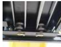
The structure of cable and pulley under main runway.
